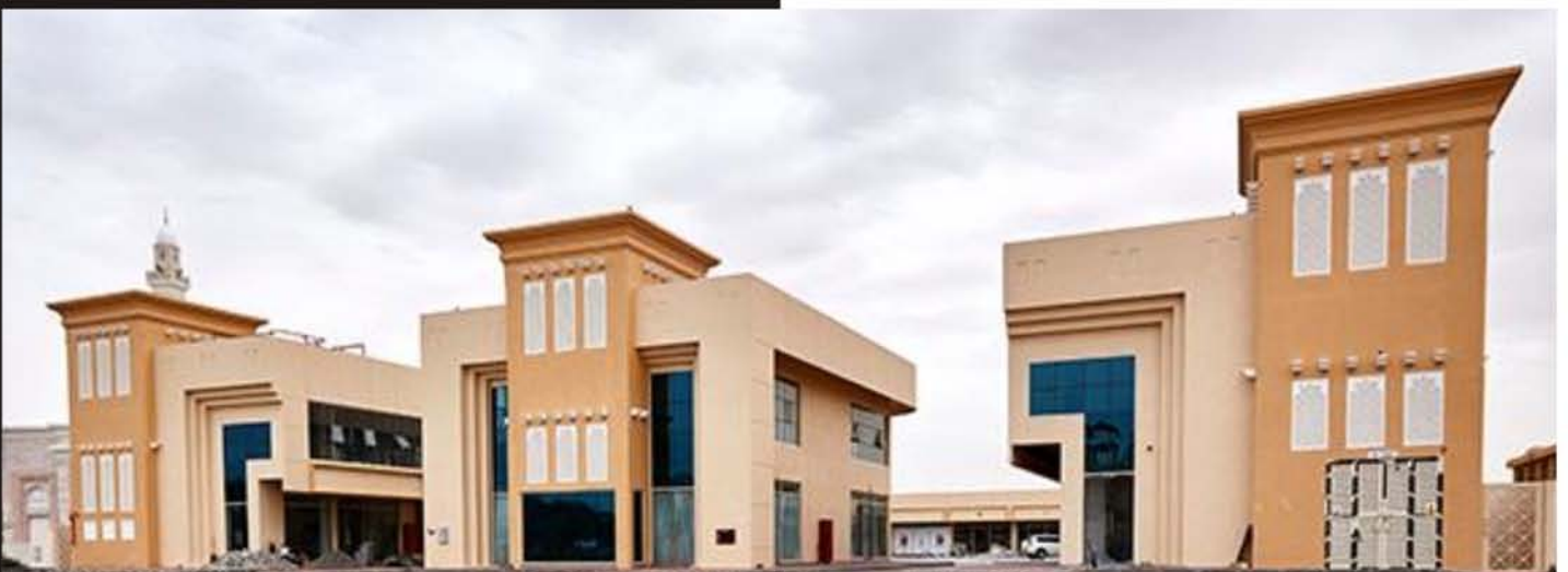
AL-Mizhar Shopping Center - Dubai, UAE
